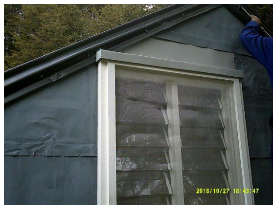
Window meshed and flashed
