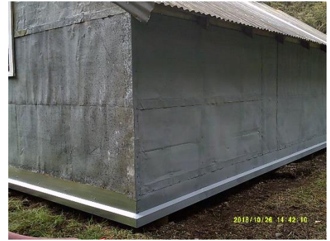
Flashing in place.
