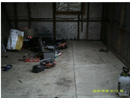
New floor laid
