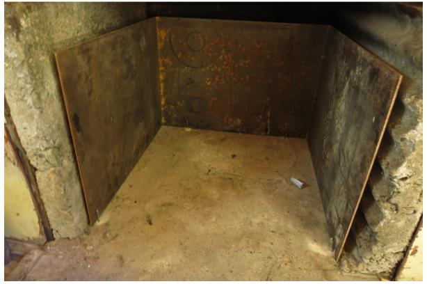
A steel insert was also placed in the fireplace to protect the crumbling concrete form further decay. A cap was made for the chimney top and a flashing installed to catch leaves between the roof and chimney.
